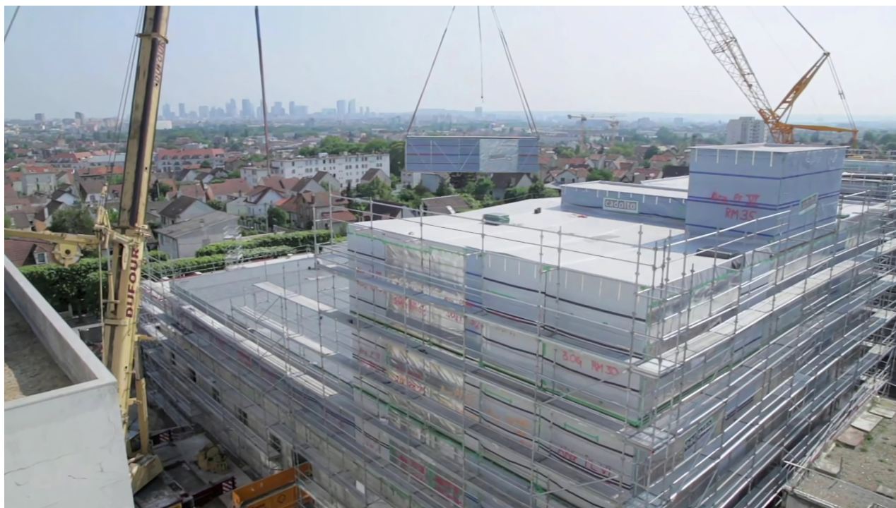
Installation des modules (Source Cadolto/GTM/BSA/Egis)
