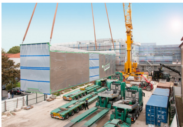
Installation des modules (Source Cadolto/GTM/BSA/Egis)
