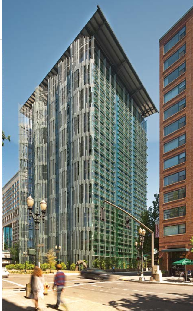
◀ The renovated Edith Green-Wendell Wyatt Federal Building is shown in its setting in Portland, Oregon.
